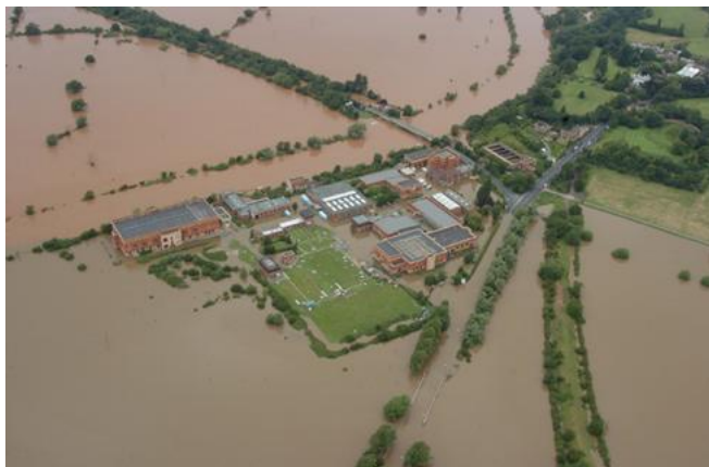
Figure 1 – Mythe Water Treatment Works under flood (source, Severn Trent Water)
