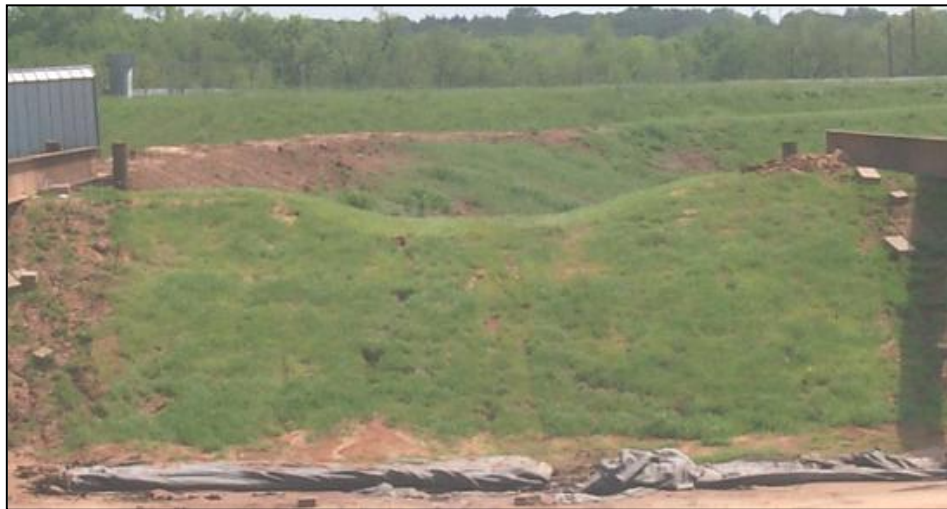
Figure 7-2: Test case 1 embankment
