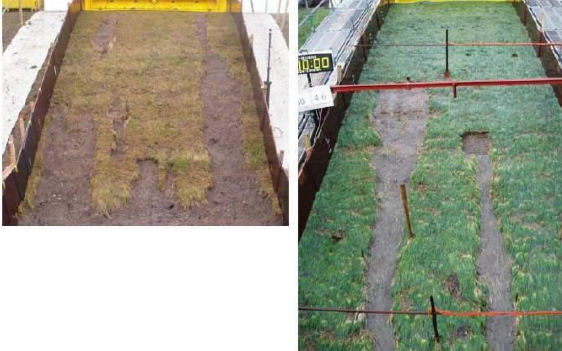
Figure 6-14: Extension of initial damage in gullies. Progress of erosion in depth was often limited and in these cases, no failure of the top layer occurred.
