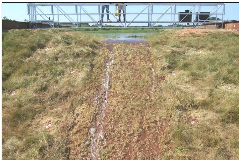
Figure 7-4: Test Case 2 embankment
