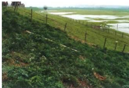
Figure 6-3: Rough herbage, severe decrease in erosion resistance (TAW 1999)
