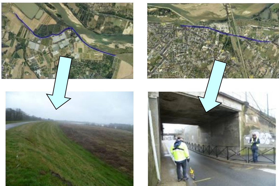
Figure 2.3 Examples of embankment levees protecting urban areas (Orléans, France). Some stretches are very lightly embedded (left side views) whereas others are very strongly embedded (right side views) in the urban environment. (© CETE Normandie Centre, DREAL Centre).
