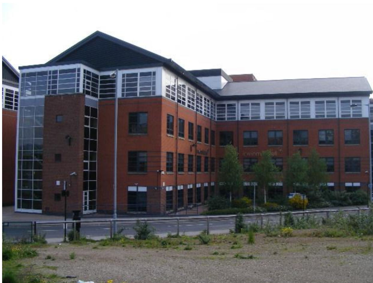
Figure 8 Case study 2, 4 storey office building
