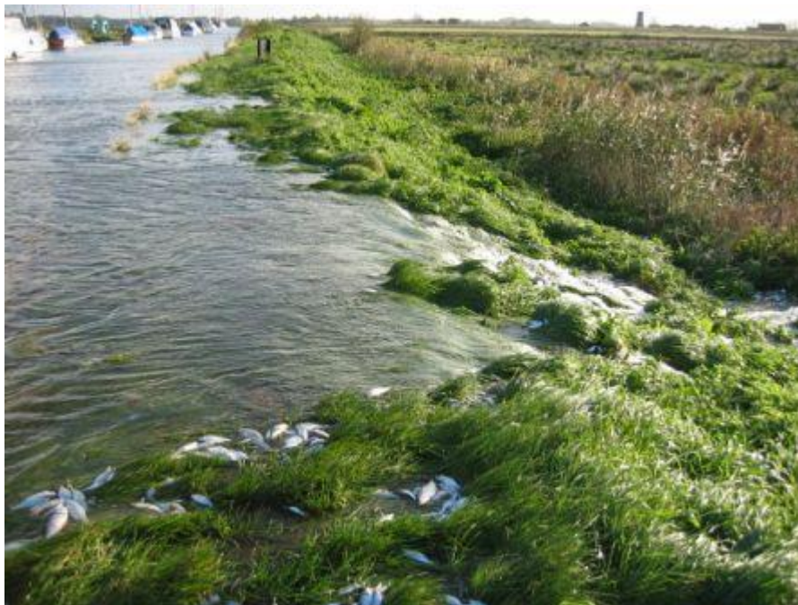
Figure 7. Overtopping grass covered flood defence (Photo courtesy HR Wallingford)
