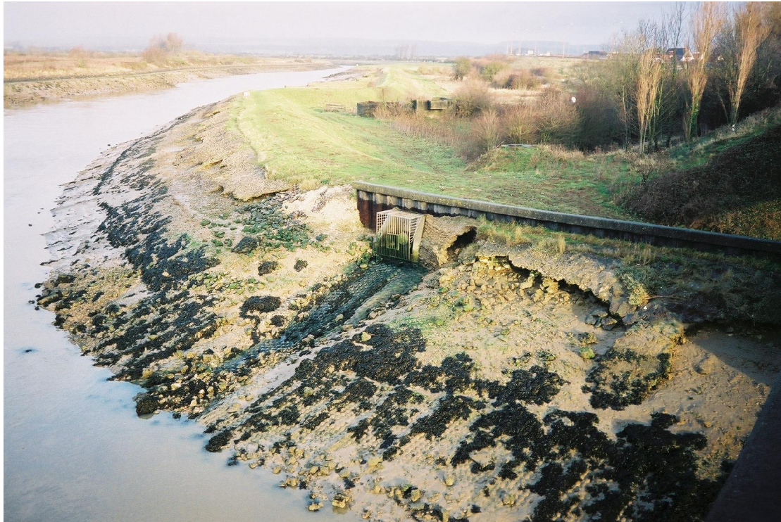
Figure 6. Structure transition in flood defence (Photo courtesy HR Wallingford)
