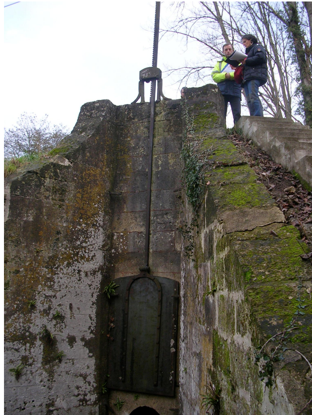
Figure 5. A culvert through a levee (Photo courtesy Cemagref)
