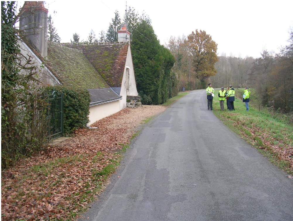
Figure 4. A house in a levee (Photo courtesy Cemagref)
