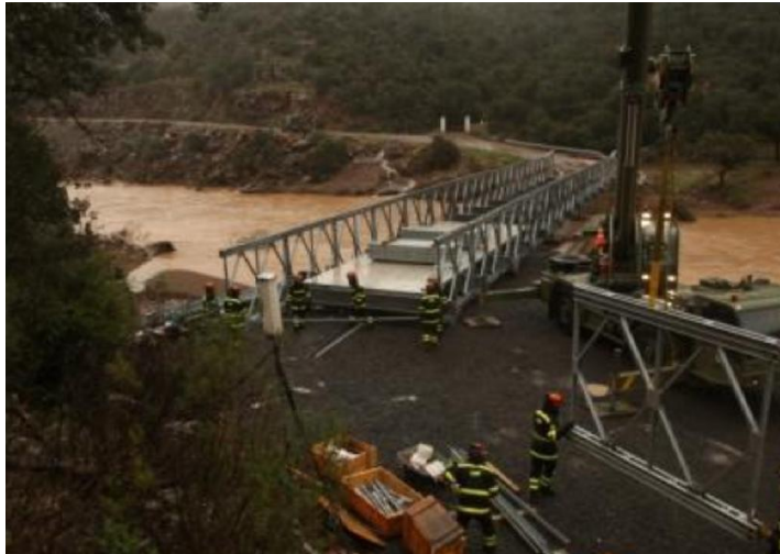
Figure 18 Military bridge assemblage
