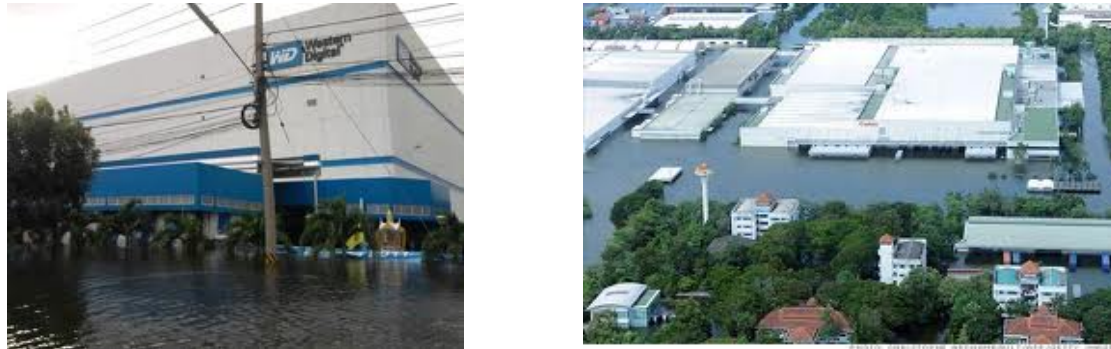
Figure 35 Details of the effect of floods in industrial infrastructure zones, Asia - 2011
