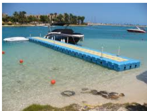
Figure 22 Floating box applied in a private marina
