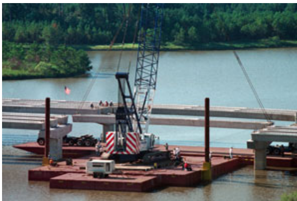
Figure 11 Examples of floating bases application
