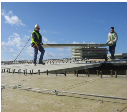
Figure 27 Construction of a composite materials lightweight bridge.
