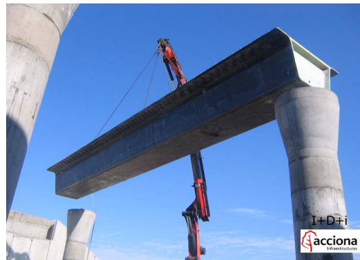
Figure 27 Construction of a composite materials lightweight bridge.
