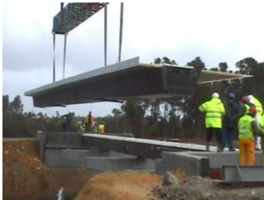
Figure 2 Lightweight bridge placements by ACCIONA, Asturias - Spain, 2004.
