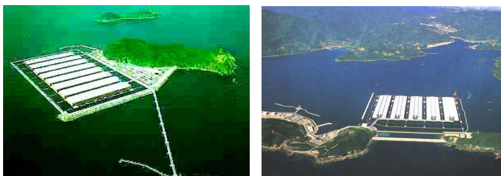
Figure 3 On the left Shirashima Floating Oil Storage Base, and on the right Kamigoto Floating Oil Storage, Japan.
