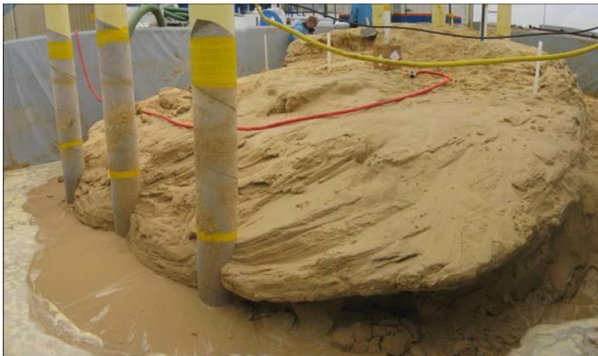
Figure 4 40 m 3 of biocemented sand strengthened with the BioGrout process
