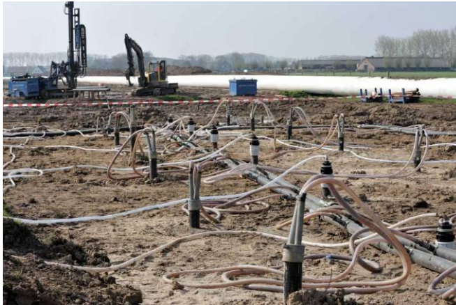
Figure 5 Cementing gravel for the horizontal drilling pilot near Nijmegen 2010.
