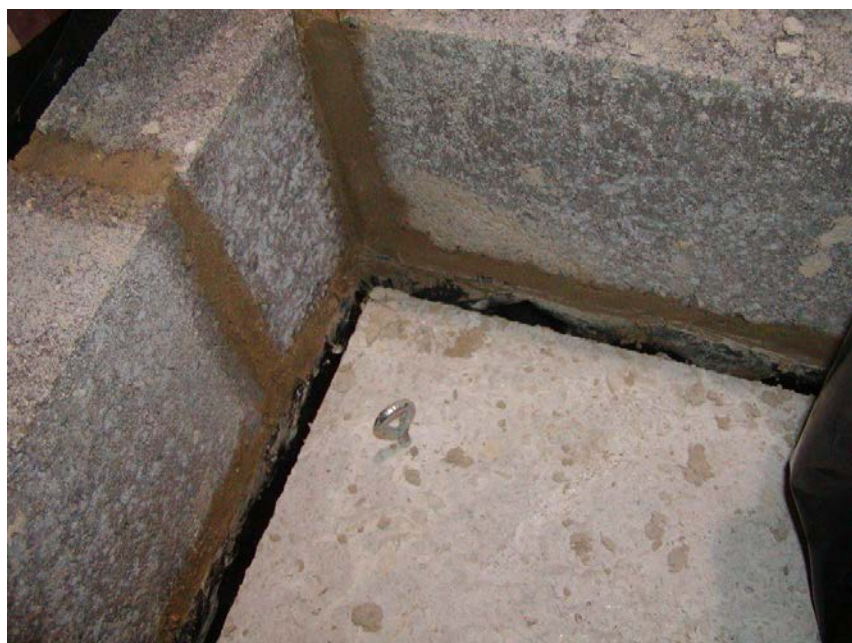
Figure 3.1 Test slab and adjacent corner wall
