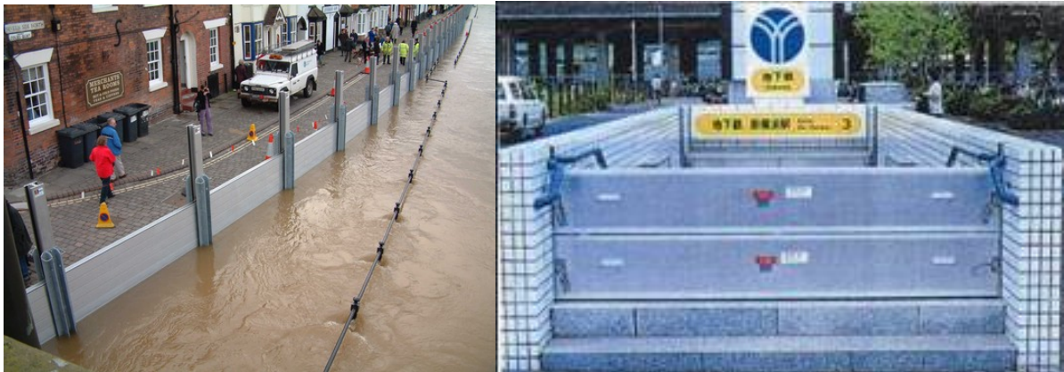
Figure 2.11: Temporary barrier, Bewdley (UK) (Singletrackworld.com, 2011); Figure 2.12: Temporary barrier at metro entrance, Tokyo (JP) (TU Delft, 2011)
