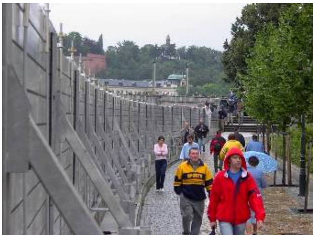
Figure 2.13: Temporary barriers in Prague (CZE) (VRV company, 2007)
