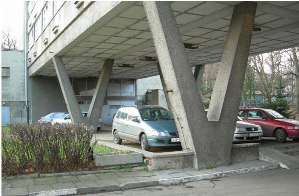
Figure 3.2 Public building built on reinforced concrete pillars, Poland
